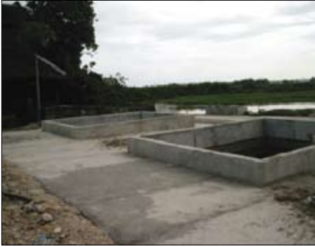
Sludge and Water Separator: Sludge from the bottom of the digester tanks is fed to a sludge collection system for dewatering. The supernatant water is fed back to the digester tank in the top zone. The dried sludge from the sludge tank is removed for fertilizer production.
